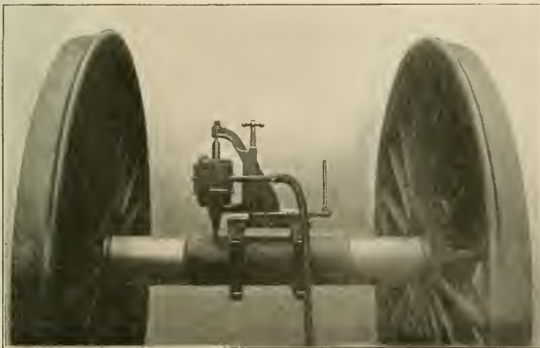
PORTABLE COTTER DRILL FOR CUTTING KEYWAYS.
